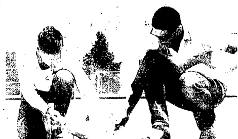
EAVERNE (left) AND RICH BROWN fill the expansion joints in the Wayne swimming pool floor, with a calking compound Sunday afternoon. The pool was filled Tuesday and all that remains is for the water to be cleaned for the opening Saturday. Rich Brown is the pool manager.
